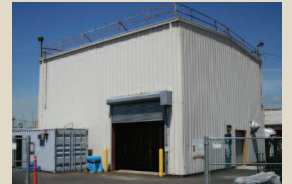
Exterior view of water treatment plant.
