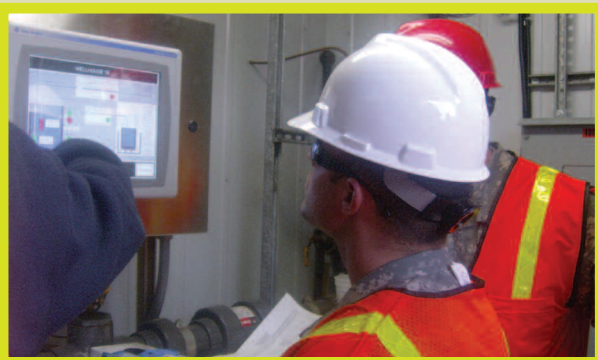
Visiting cadets study a display of system controls and recovery tank levels for the groundwater pump, product pump, product tank and sensors in a product recovery well.
